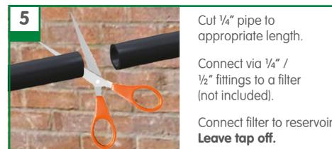
Cut ¼" pipe to appropriate length. Connect via ¼" / ½" fittings to a filter (not included). Connect filter to reservoir. **Leave tap off.**
