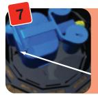
Once you have connected the AQUAvalve5 to the 3/8" pipe, simply pull the pipe back through the 3/8" Top Hat Grommet, so that all the excess pipe inside the AQUAbox Spyder is pulled out. As you pull the pipe out lower the AQUAvalve5 so that it locates onto the Tee section in the AQUAbox Spyder.
